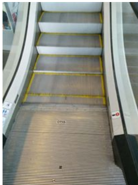
Lack of clear differentiation between steps is confusing and dangerous for someone with cognitive or visual impairment.
