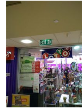
Blocked exit signage could hinder escape during an emergency.
